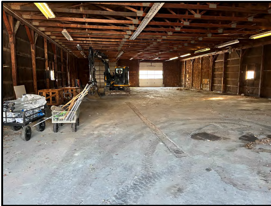
SUBJECT BUILDING INTERIOR GARAGE AND STORAGE AREA WITH TRENCH DRAIN
