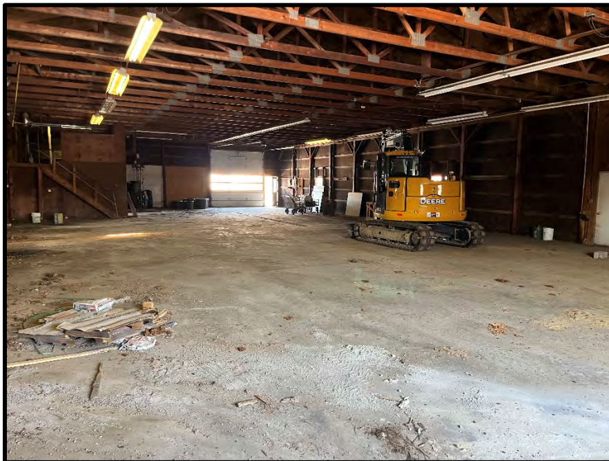
SUBJECT BUILDING INTERIOR GARAGE AND STORAGE AREA
