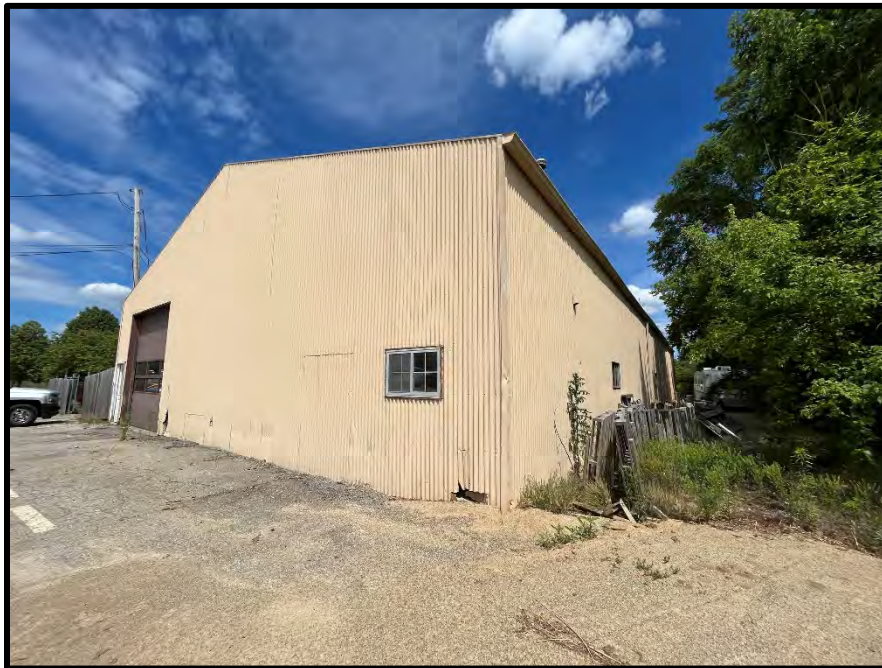
SUBJECT BUILDING – FACING NORTHEAST
