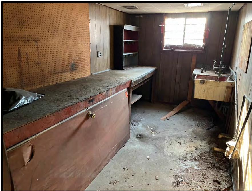
SUBJECT BUILDING INTERIOR STORAGE ROOM
