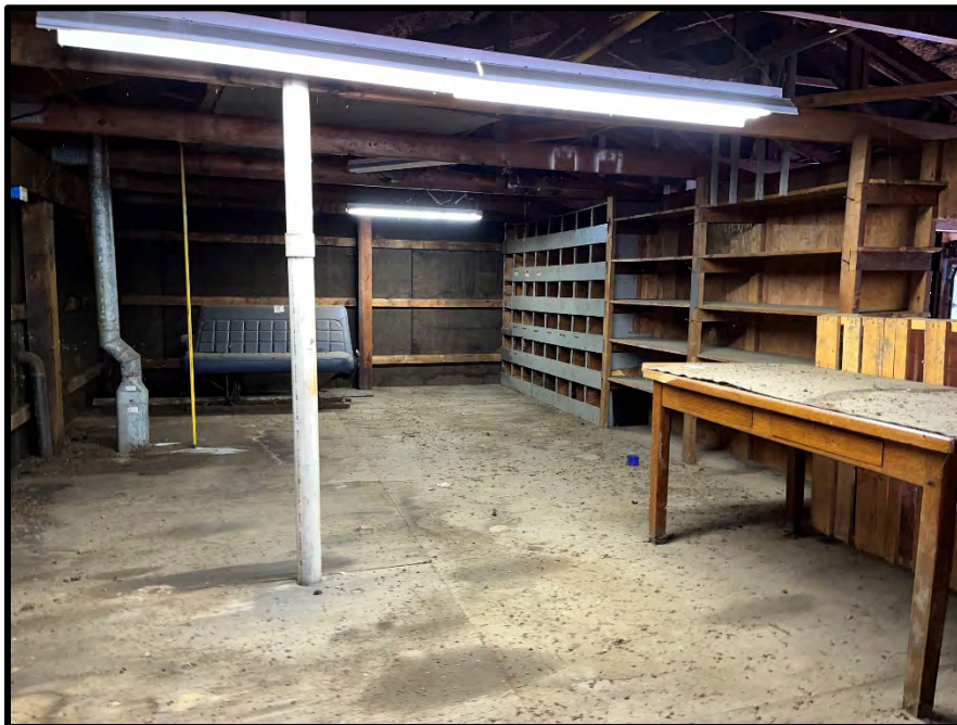
SUBJECT BUILDING INTERIOR MEZZAINE STORAGE AREA
