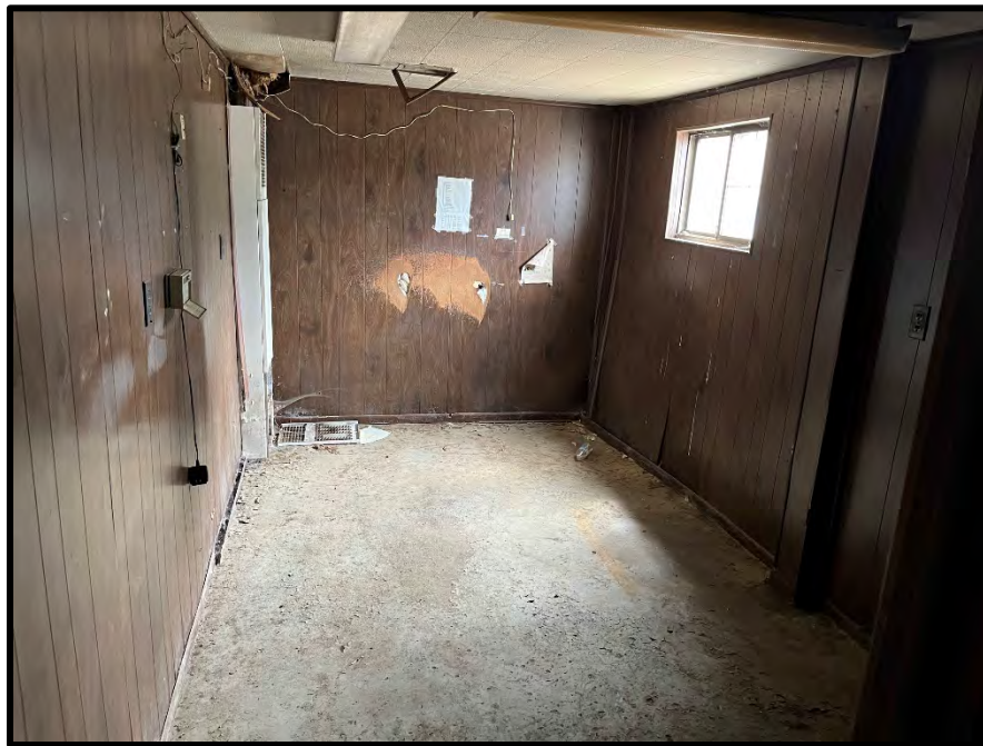
SUBJECT BUILDING INTERIOR OFFICE AREA
