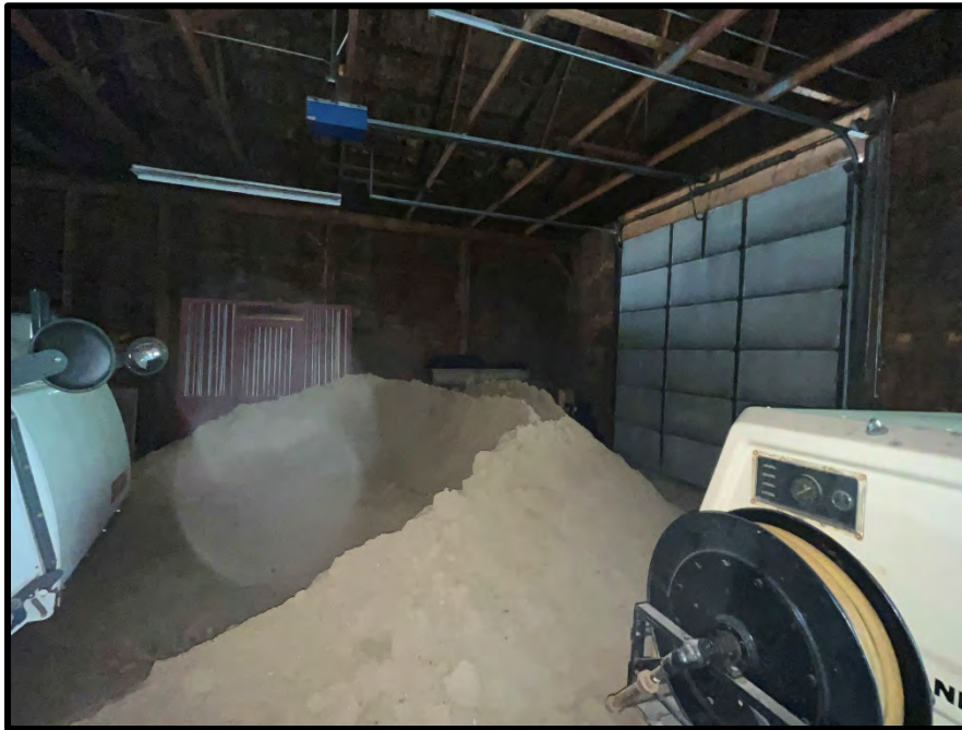
VIEW OF SAND PILE IN THE EASTERN PORTION OF SUBJECT BUILDING
