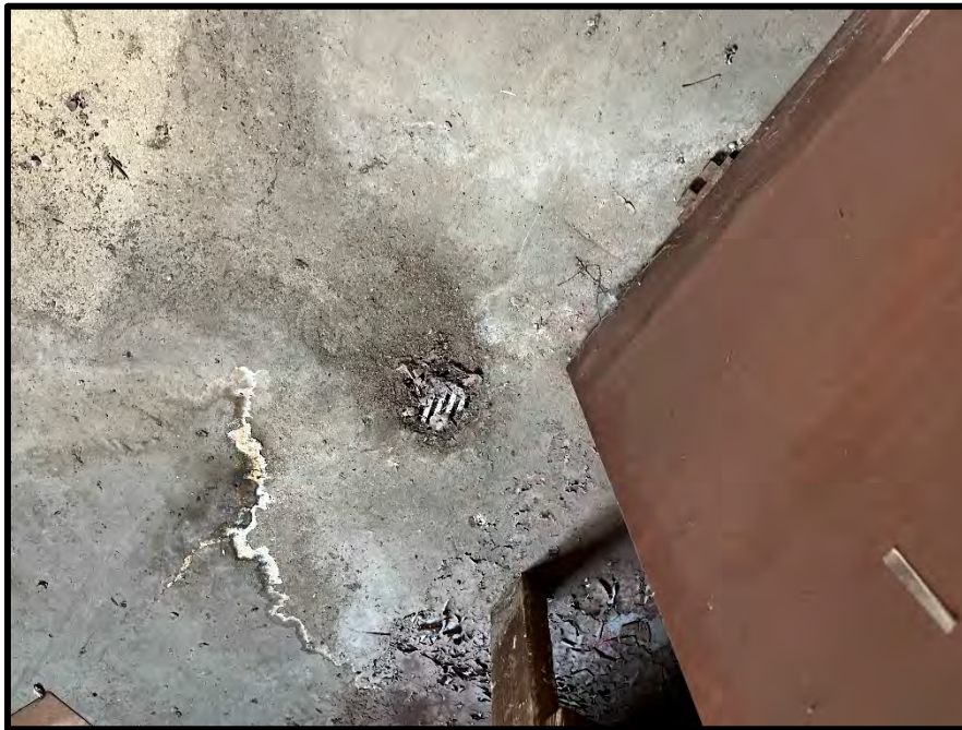
VIEW OF FLOOR DRAIN LOCATED IN SOUTHWESTERN PORTION OF SUBJECT BUILDING
