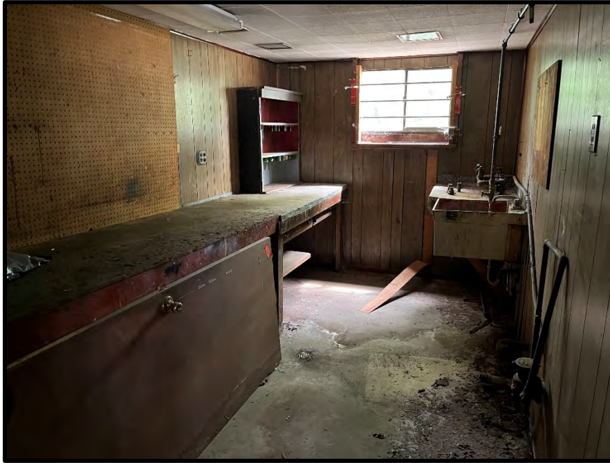
SUBJECT BUILDING INTERIOR STORAGE ROOM
