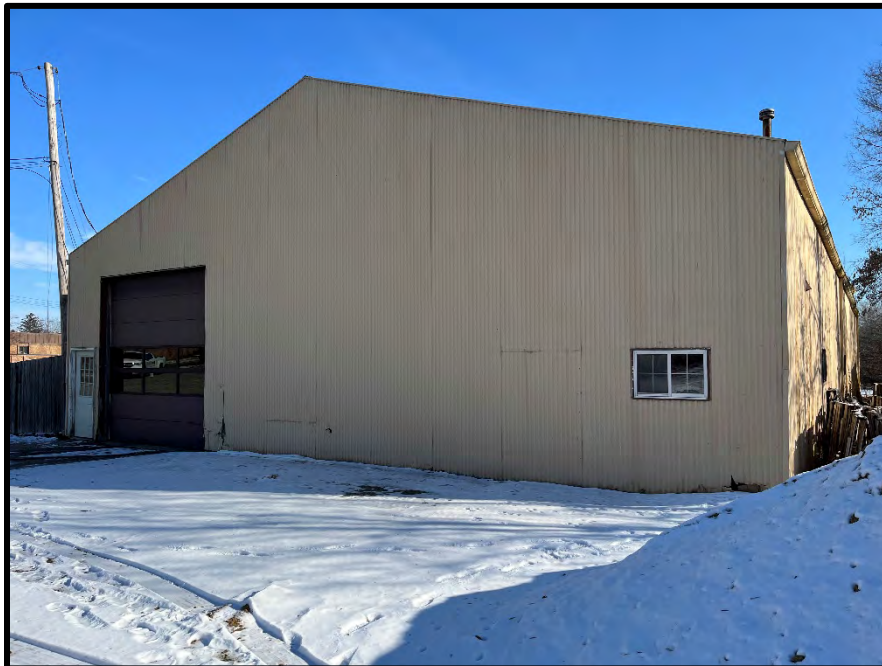
SUBJECT BUILDING – FACING NORTHEAST
